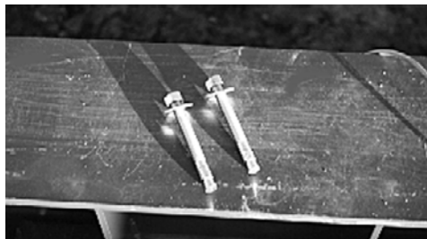
Figure 4-9. Anchor Bolts with Washers
