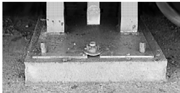
Figure 4-13. Completed Baseplate Grouting
