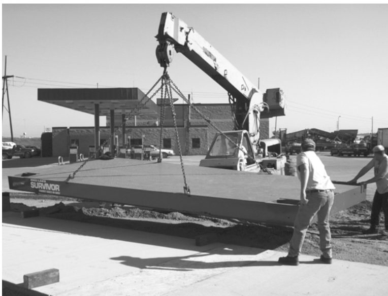
Figure 2-1. Lifting Deck Modules (Steel Deck)
