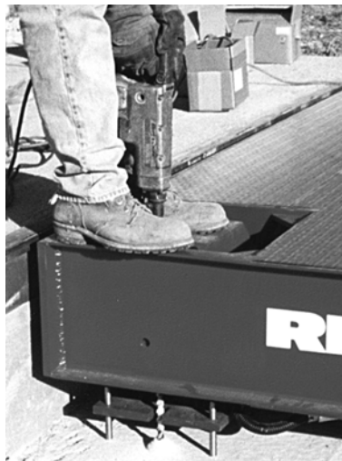
Figure 4-8. Drill Anchor Bolt Holes
